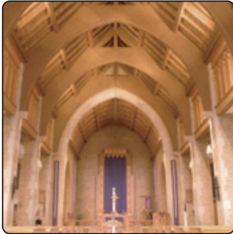
Stone walls, columns and majestic wooden arches create acoustical challenges.
